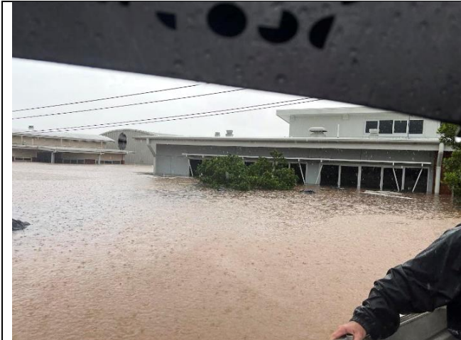
The new TAS building only completed two years ago. The flood of this building is 12.5m above normal river level.
