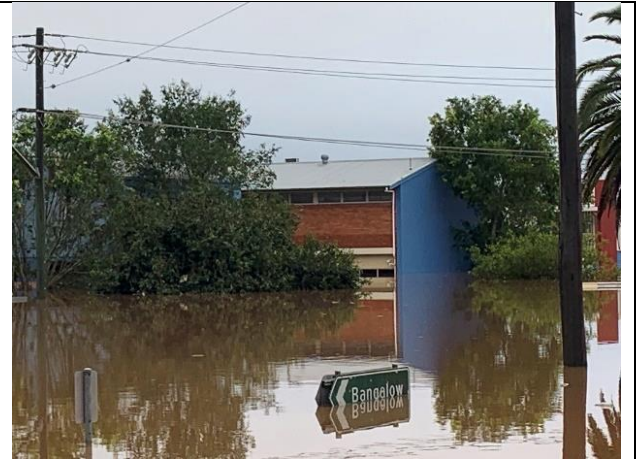
You can see the peak water level line on this building. This is on the first floor of the St Joseph's Site.
