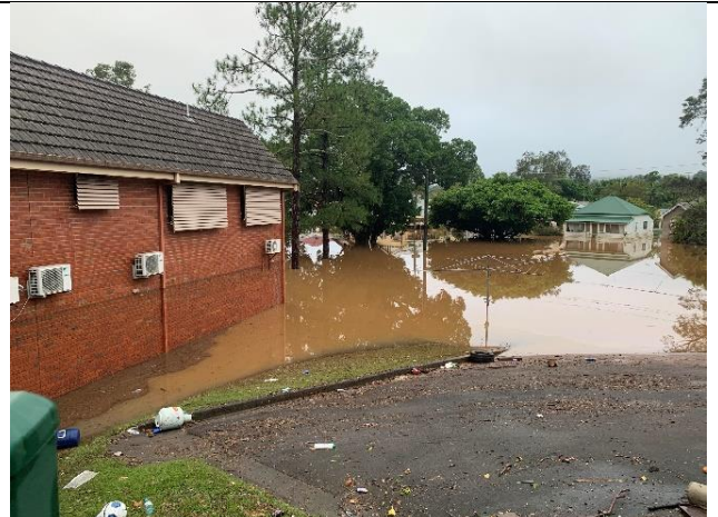
The flood level line on the side of the presbytery.
