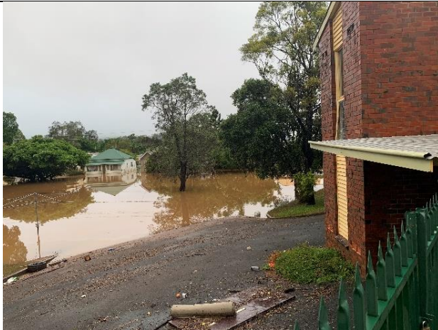
Debris at the carport entry of the Brothers' House
