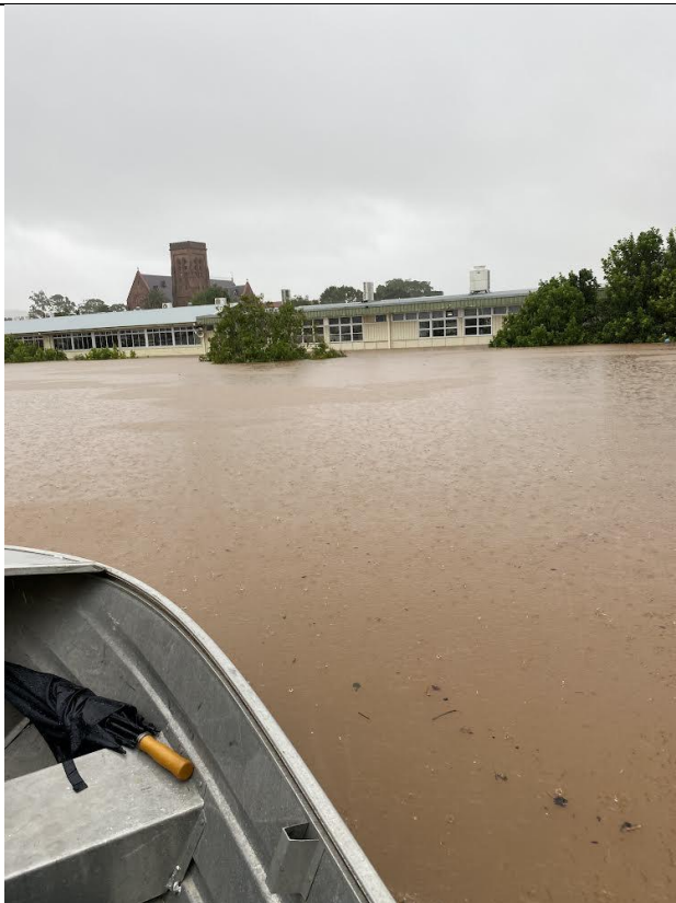
The main building on the St Joseph's Site. You can clearly see the water has well and truly entered the first floor.
